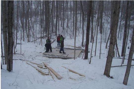
Building a new bridge in Duanesburg...
